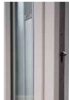
Multi-Point Locking System on Venting Sidelite
